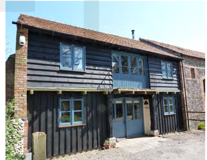
Barn conversion on Binham Lane
