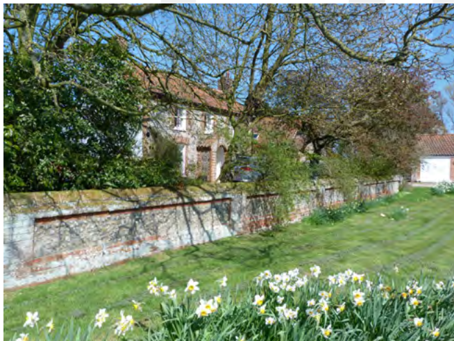
Brick and flint wall to the south of Church Farm House
